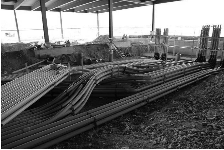
Figure 3.1.2: Underground PVC Conduit in Data Center Construction
